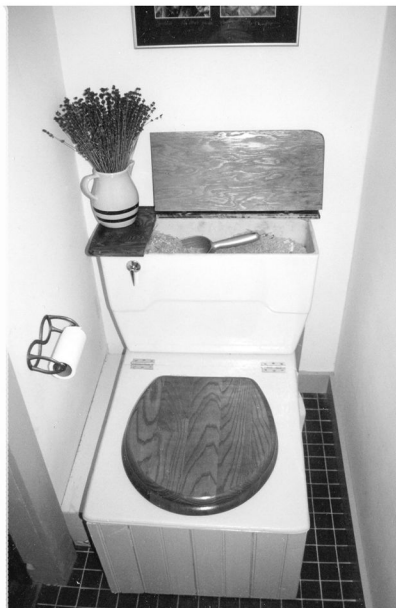
use of old toilet tank for sawdust storage
